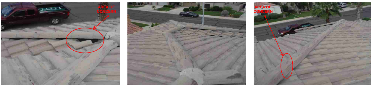
3.7 - Roof Pictures Continued
