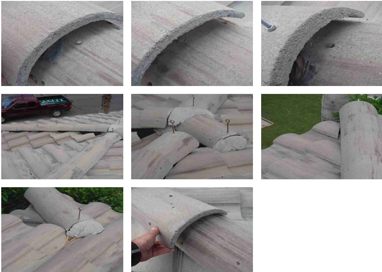
FYI 3.6 - Additional Roof Pictures Continued
